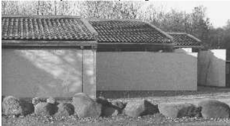
Figure 5 View from street Utzon's 'Expansiva' 1969 at Hellebaek Source Utzon and the New Tradition 2004:177
