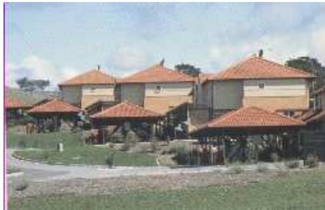
Figure 15 Repetition to form streetscape Rex Addison's Development at Kambah, Canberra. Figure Australian Architects 5:30
