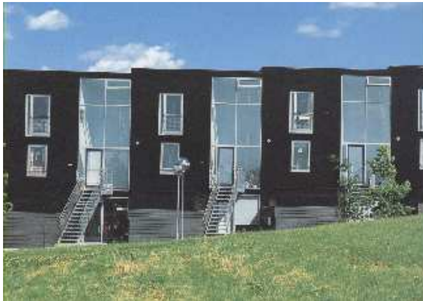
Figure 10 View of houses from street in Egebjerggaard, Tegnestuen Vandkunsten Denmark Source Bo i By exhibition catalogue 1996:44
